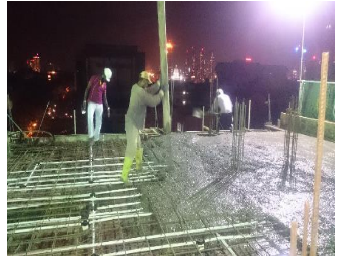
Figure 2– 04 th floor slab conduiting
