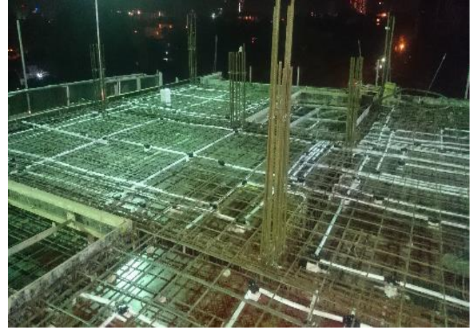
Figure 2– 04 th floor slab conduiting
