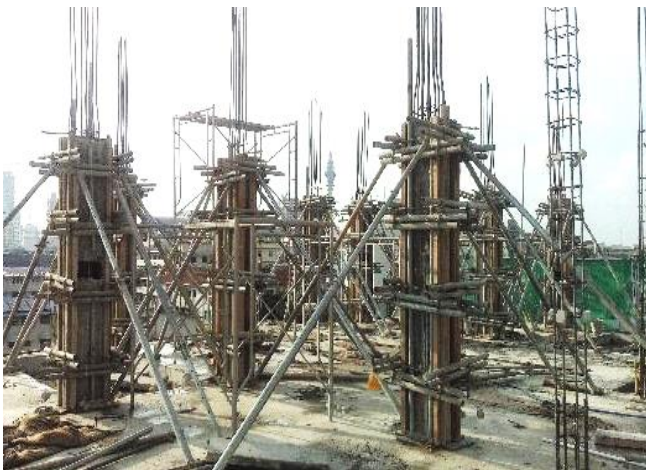
Figure 9 – 04 th to 05 th floor Lift well RF work
