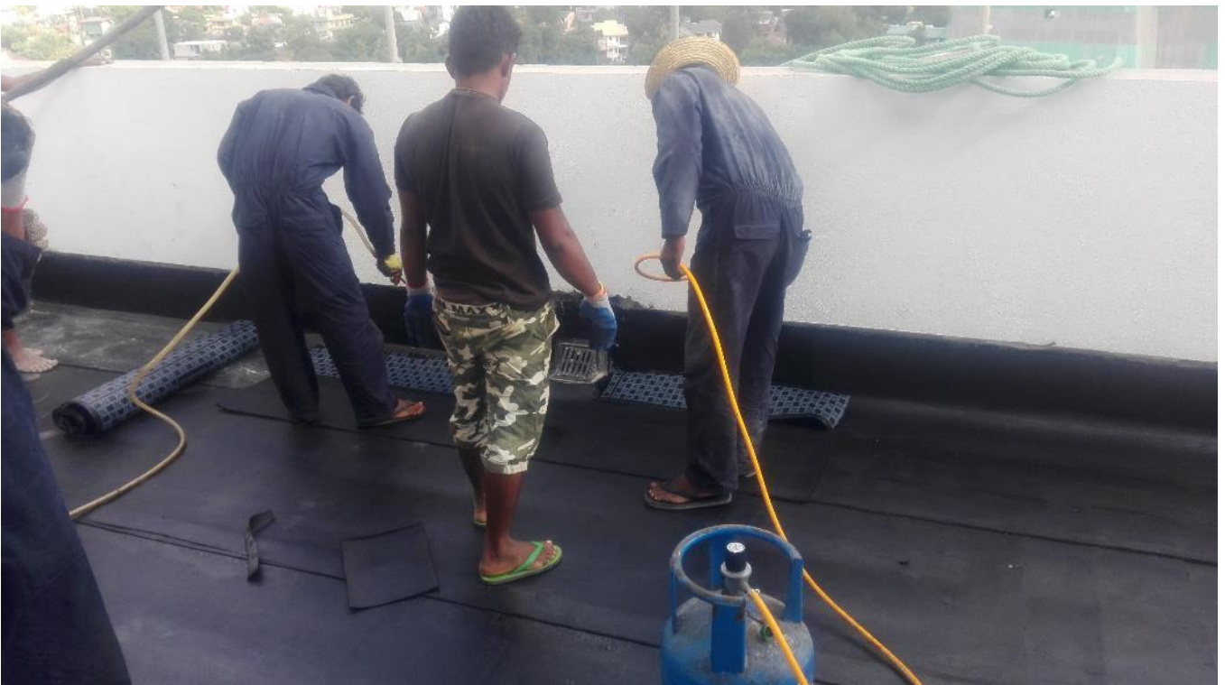
Figure.10 – Roof Terrace Waterproofing
