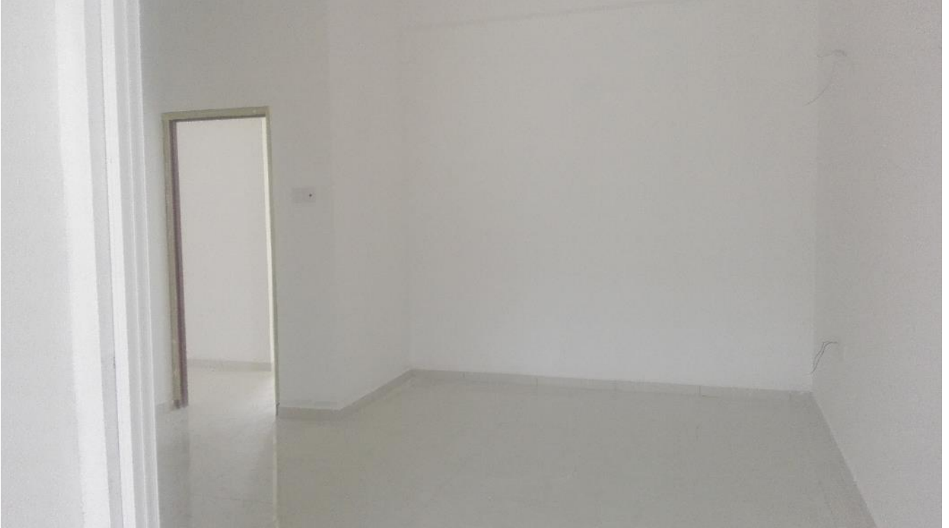
Figure.05 – Bed Room after Initial coat of Paint
