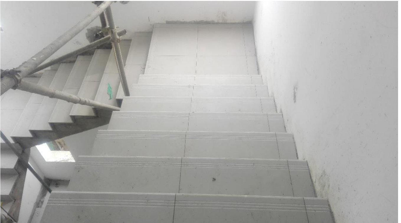
Figure.08 – Staircase Tiling
