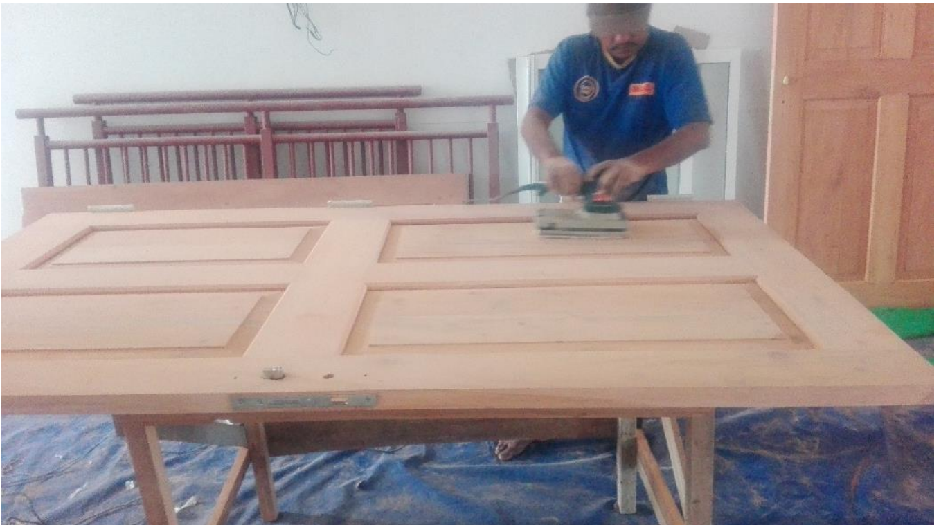
Figure.06 – Main Door Sanding
