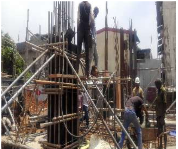
Column Concrete Works
