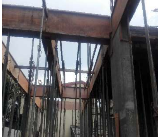
Mezzanine Floor Form Works
