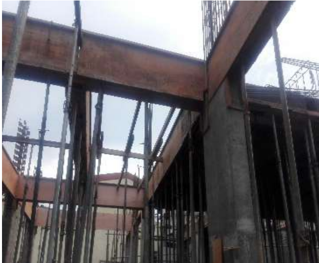
Mezzanine Floor Form Works
