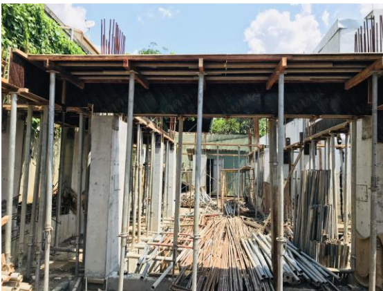
Mezzanine Floor Slab on Progress
