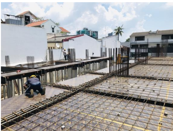
Mezzanine Floor Slab R/F Work
