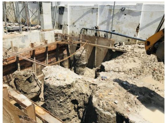
Excavation Work on Progress for Passenger Lift
