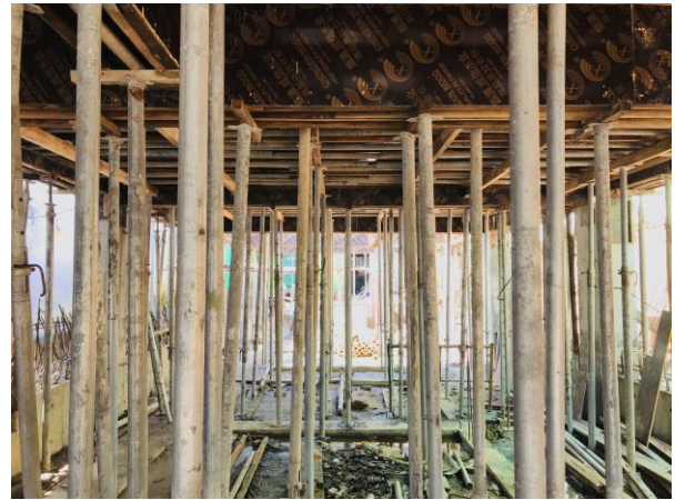
Mezzanine Floor Slab on Progress
