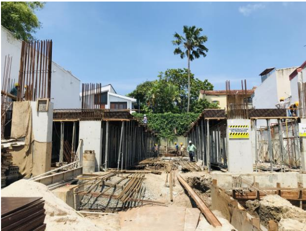
G.F. Structural Works on Progress
