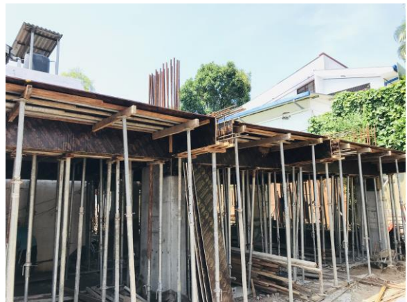
Mezzanine Floor Slab Formwork
